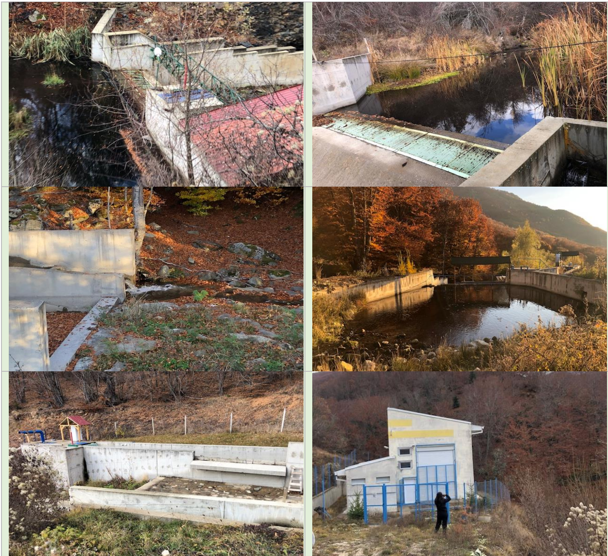
Figure 39 - 44. Near the water intake and SHPP's.
